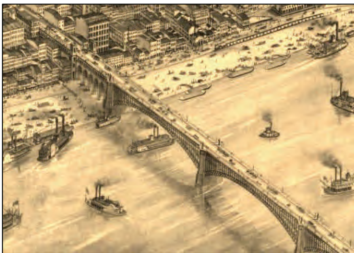
Figure 8 | Compton & Dry, Plate 2 showing the Eads Bridge.
